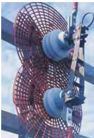
BISG-60/115-02 installed on switch
