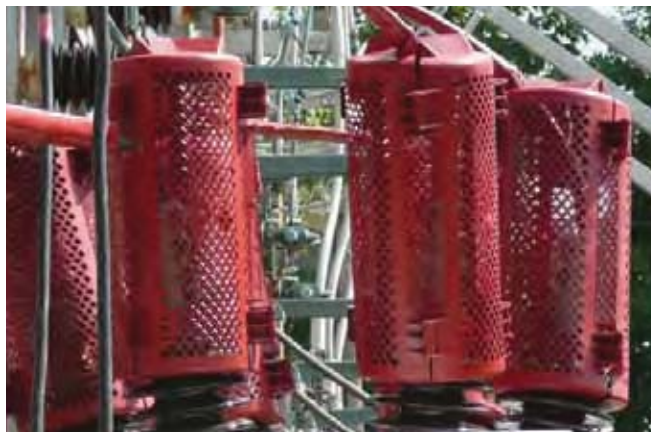
BCAC-IC Installed on Bushings
