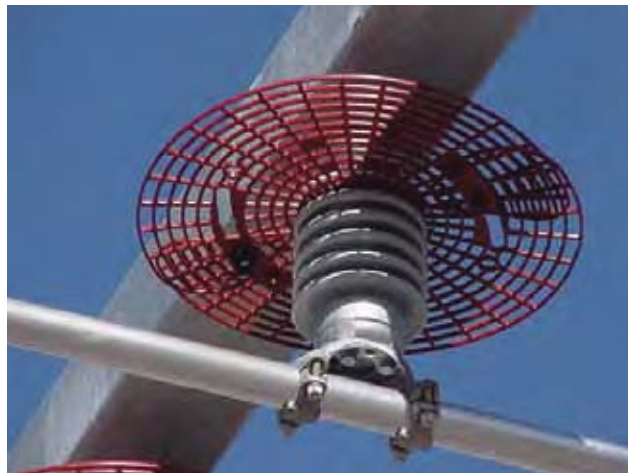
BISG-60/115-02 installed on bus support insulator
